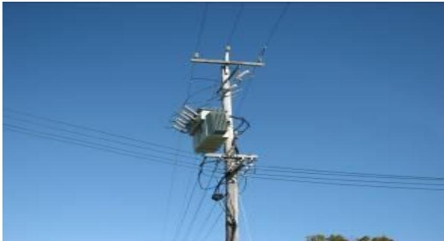
**Figure 58:** HV outdoor aerial mounted equipment
