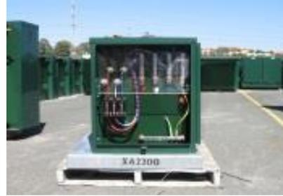
**Figure 13:** Rural/SPUD transformer supply (1 phase)
