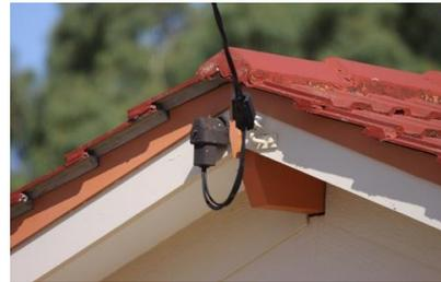
**Figure 14:** Standard overhead connection and PoA
