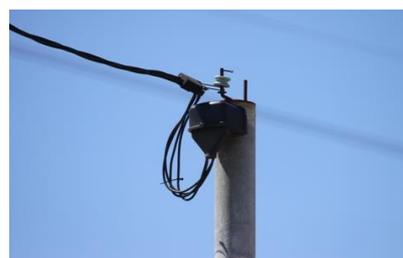
**Figure 15:** Domestic aerial service cable connection (3 phase)
