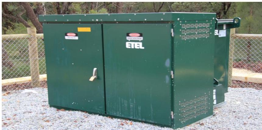
**Figure 55:** Modular package substation
