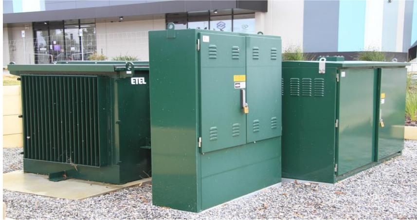
**Figure 56:** Non modular package (cluster) substation arrangement
