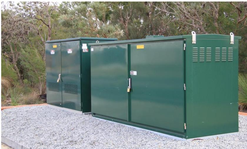
**Figure 57:** HV outdoor ground mounted switchgear & transformer
