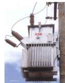
**Purpose:** This form covers the testing and commissioning requirements for new or replacement pole mounted SWER isolation transformers up to 200 kVA before energisation.
