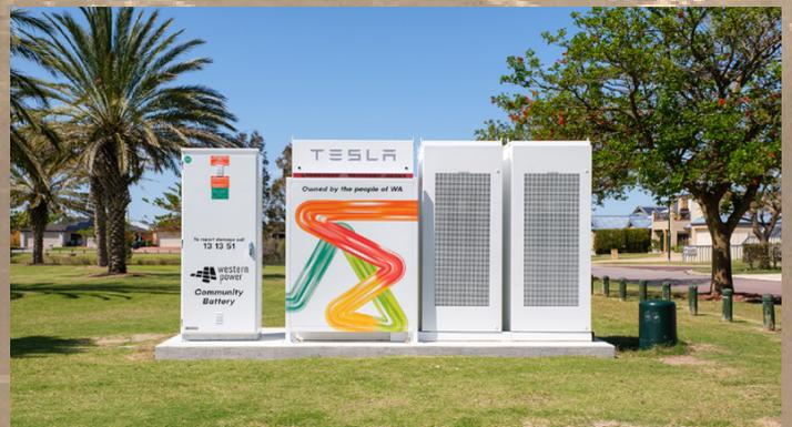
To help our transition to renewable resources, we can expect to see more batteries like this on our streets. Batteries can store the excess solar electricity made during daylight hours and release it during peak use times in the evening and early morning.
