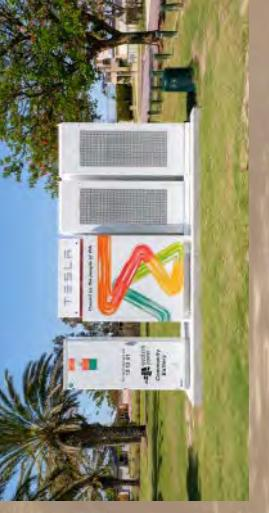
To help our transition to renewable resources, we can expect to see more batteries like this on our streets. Batteries can store the excess solar electricity made during daylight hours and release it during peak use times in the evening and early morning.
